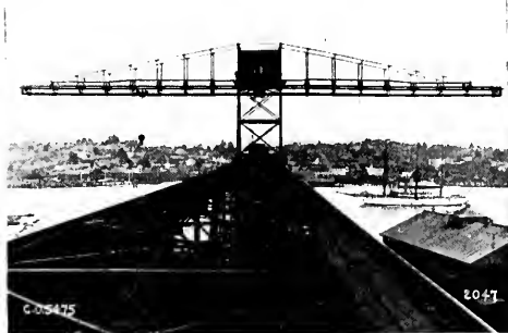
6-ton double cantilever crane at Mare Island Navy Yard.
